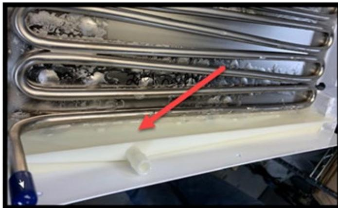
Figure 2: Drip Tray and tubing connecting point
